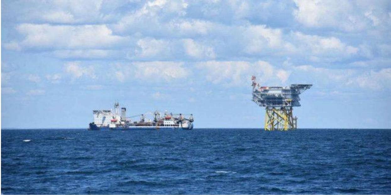
*The offshore substation that each of Vineyard Wind 1's 62 turbines will connect to (right) is seen on Aug. 1, 2023. At left is the "cable lay vessel" Giulio Verne, which connected the wind farm's export cable to the substation.*
